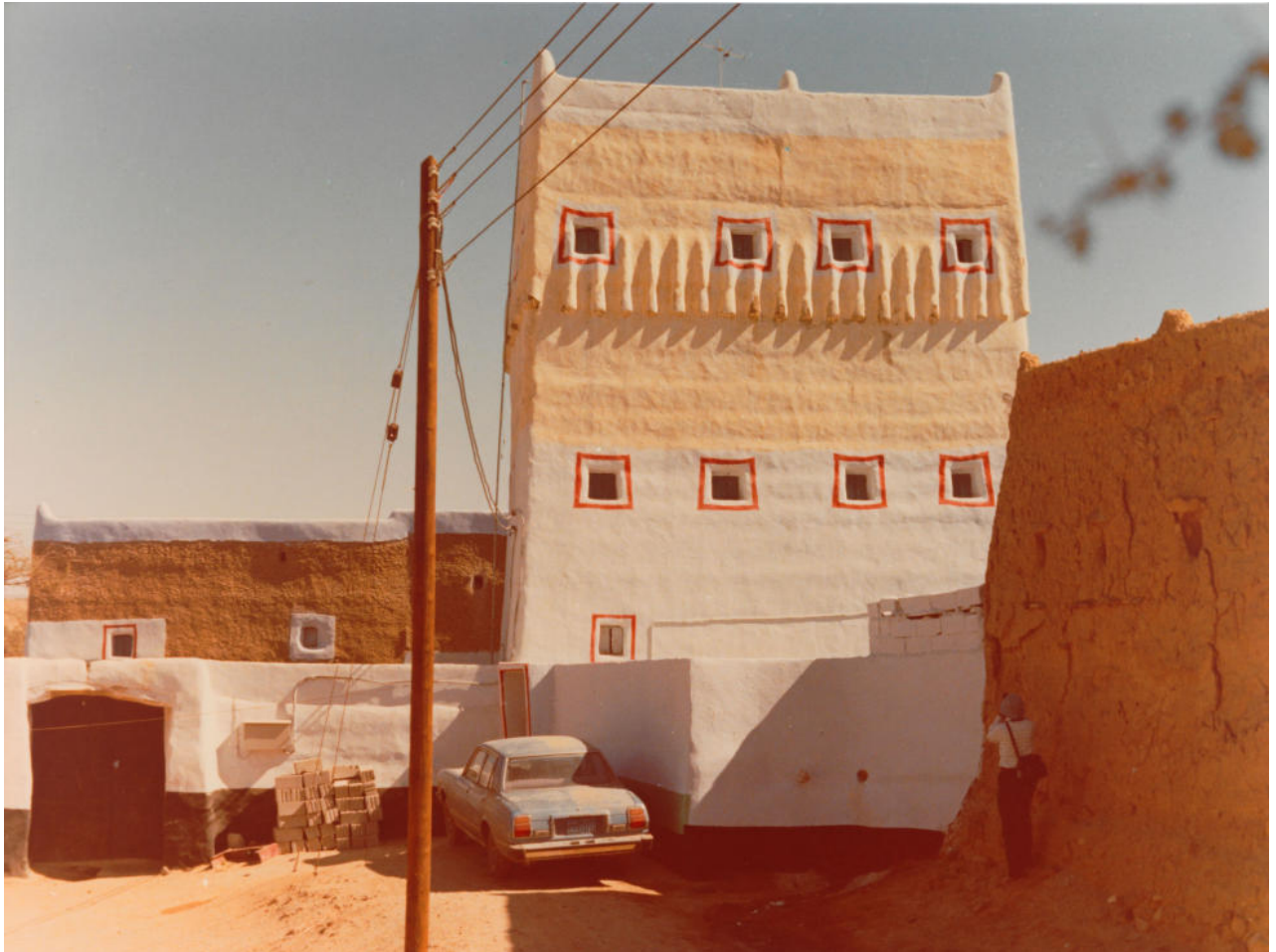
Christian Winterhalter, Traditional architectural style in the Asir region, Saudi Arabia, c. 1978
